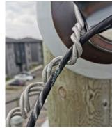
waste of power for utilities. Corona effect generates gases which are corrosive and can degrade and embrittle nearby materials.
